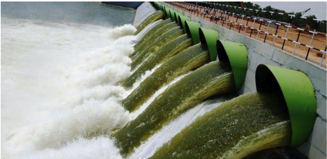
Pump of the sundilla barrage
