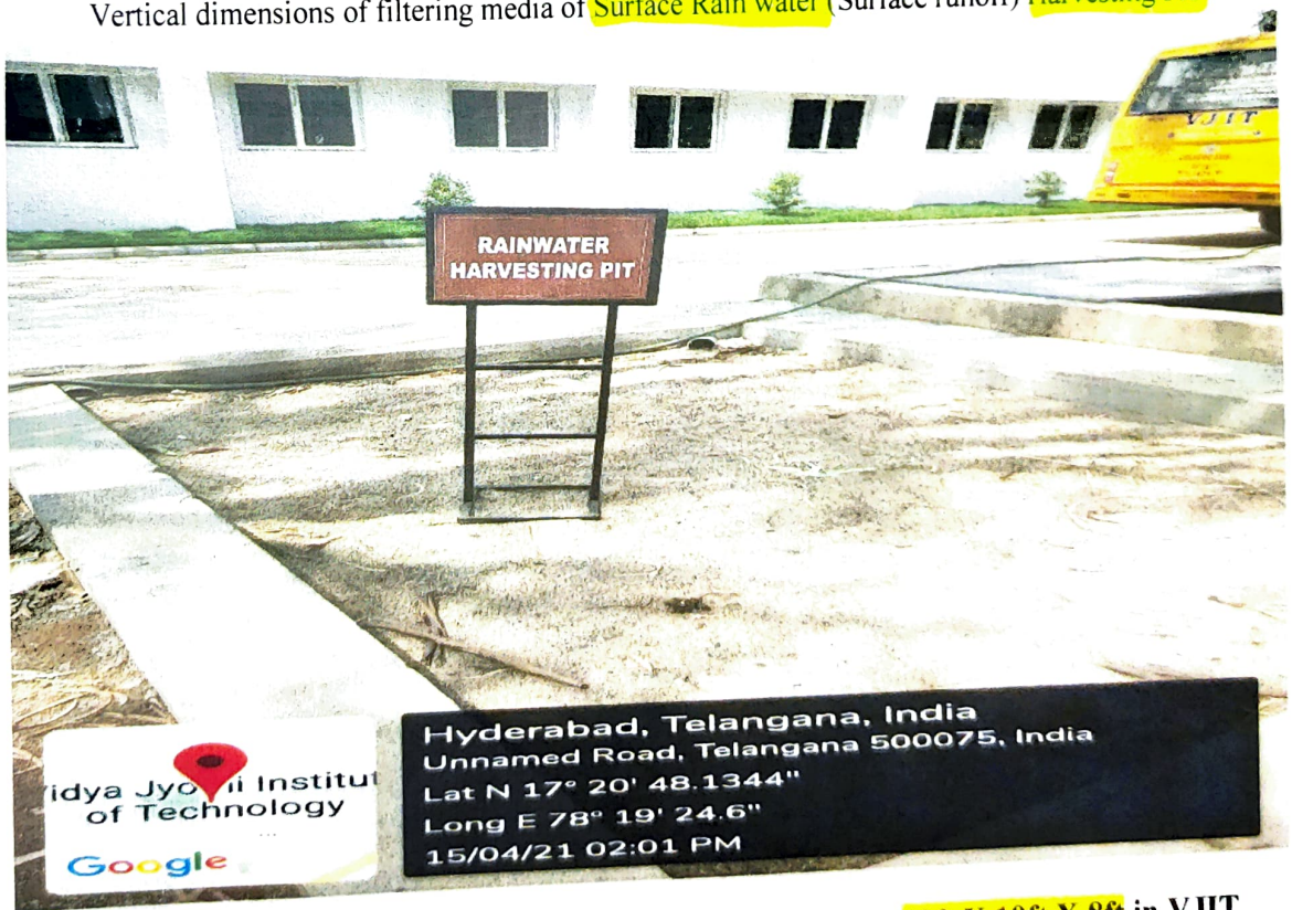
Surface Rain Water (Surface runoff) Harvesting Pit of Size 10ft X 10ft X 8ft in VJIT, Hyderabad Campus
