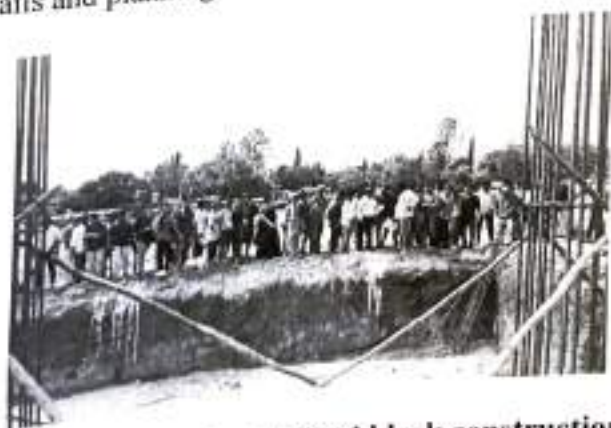
Students visited VJIT new hostel block construction Site
