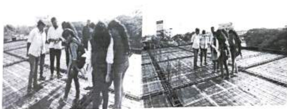
Field visit on the topic Arrangement of Steel bars
